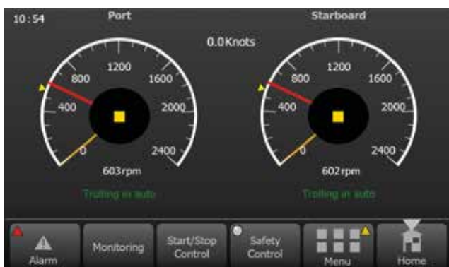
Fig. 11b: Home screen – twin high-speed engine plant
