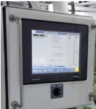
Fig. 54: Cabinet with local operator panel for propeller (LOP-P) – placed on four-stroke engine
